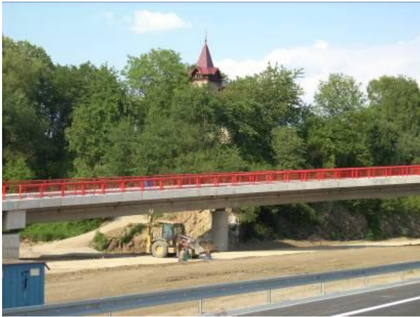
Figure 6: Highway in construction: strong environmental impact (Corridor 5 - Povaska Bystrica - Zilina line)
